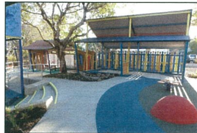
3. Upgraded shelters and sandpit
